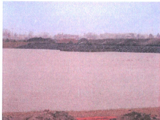
The ADF Pond detains stormwater at the Base Western Perimeter before passing through a controlled outflow structure into the City of Aurora.
