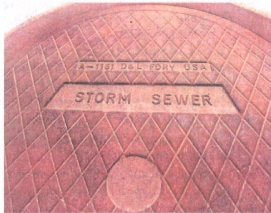
All manholes on the Buckley AFB storm water system shall be marked "Storm Sewer"
