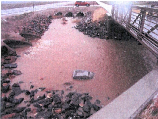
Over 600 acres of surface drainage converge at this single point, flowing under the pedestrian bridge into the ADF Detention Pond.
