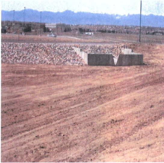
The Industrial Valley Detention Pond collects stormwater from a 300 acre area with capacity to control outflow from a 100-year flood event.
